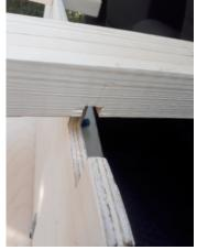
The middle lath is fastened to an alternative piece of board with bolts – and with a piece of wood between the board and the lath to give the correct hight.
